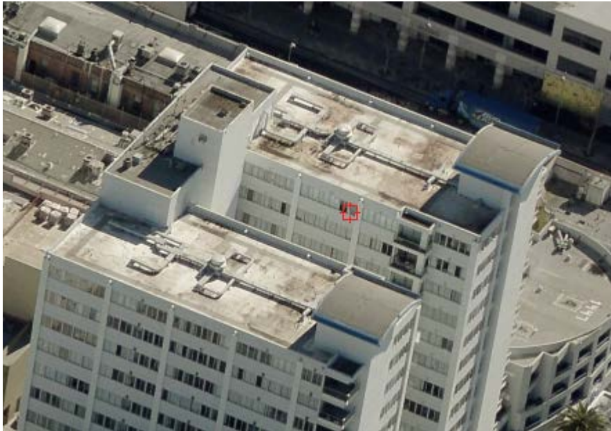
Figure 45. Rooftop of Pacific Plaza Building
