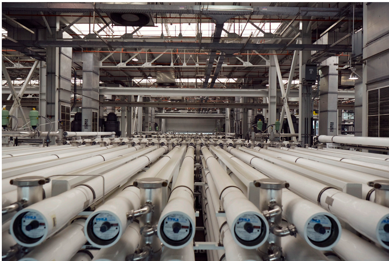
Reverse osmosis units at the Orange County Water District's Groundwater Replenishment System plant. (photo credit: Orange County Water District).
