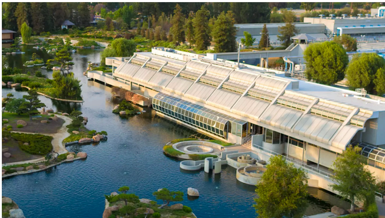
Aerial view of the Donald C. Tillman Water Reclamation Plant in Los Angeles. (photo credit: L.A. Sanitation and Environment).
