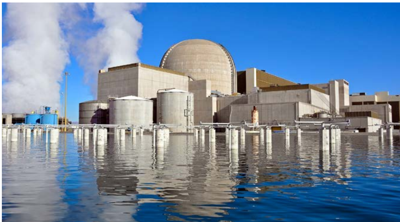
The Palo Verde Generating Station near Tonopah, Arizona. (photo credit: photo from LinkedIn).
