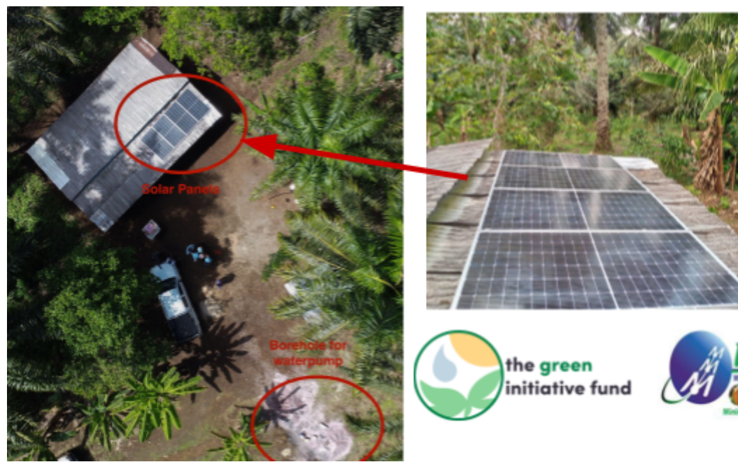
Figure 14 Solar panel installation.
